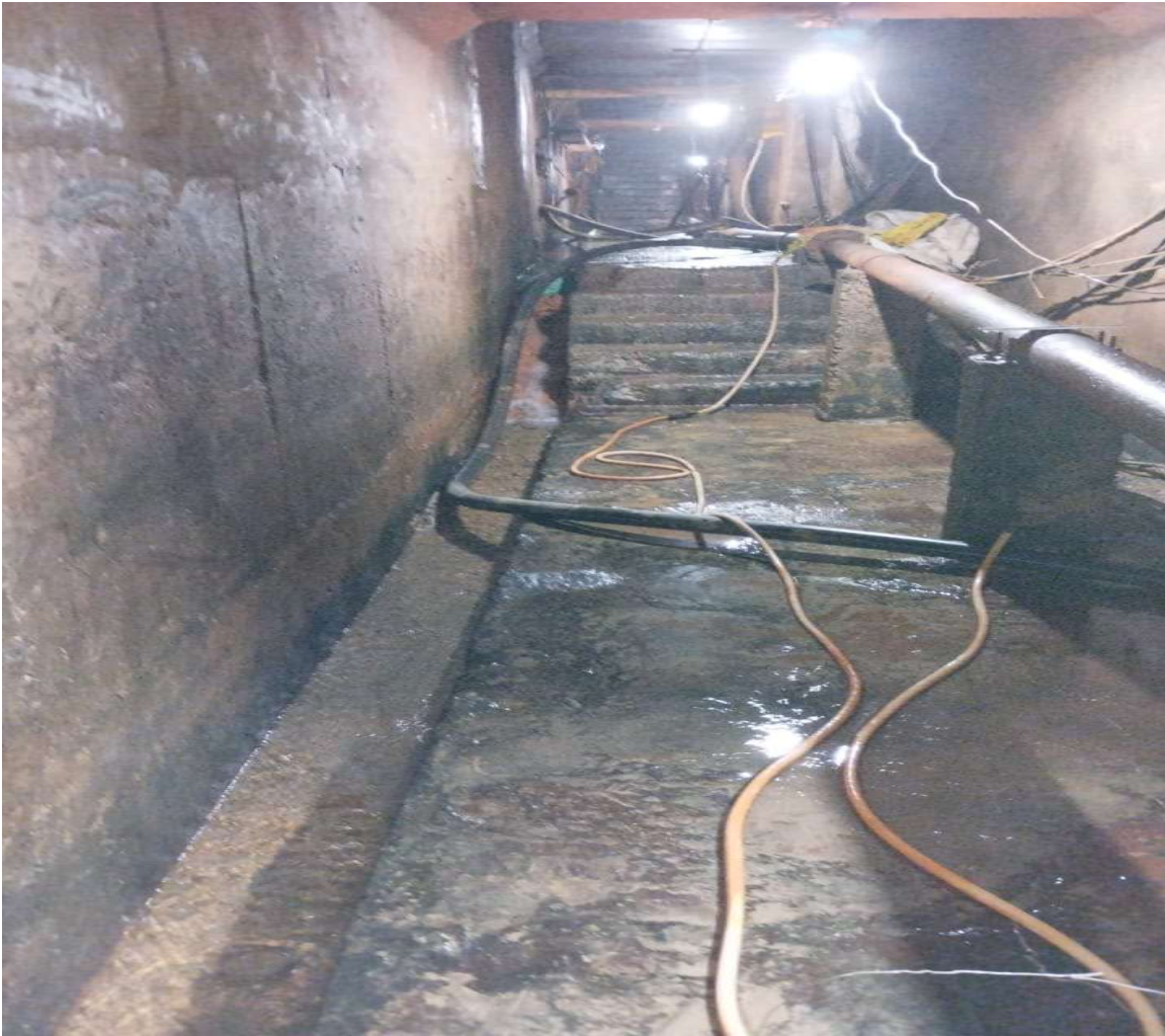
Dam gallery of Hatidubi dam, KLHEP
